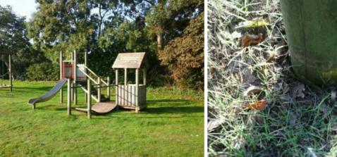
Finding: There is some strimmer damage apparent on Action: the posts, this can penetrate the preservative applied to the timber and accelerate the rotting process
