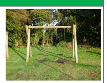
Finding 2 Finding 1 The grass mats are silted up and the soil is compacted; this may have an effect on the impact absorbing properties of the surface - Lift and relay mats or test impact absorbing properties to ensure the correct surface qualities are maintained for the equipment There are gaps opening between the grass mat tiles - Reinstate surface Finding 3 Finding 4
