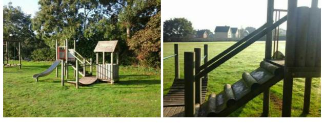
Finding: The unit is easily accessible and should have Action: the appropriate barriers installed as the height of the unit exceeds 600mm
