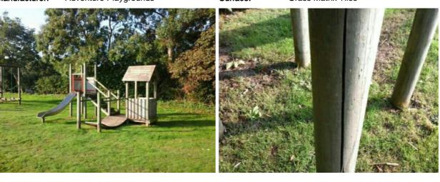
Finding: The timber has a number of air cracks apparent, the splits will have penetrated the preservative applied to the timber and allow water ingress to the unprotected areas
